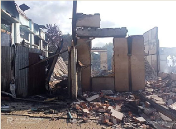
Photo - 5 A house burned down
